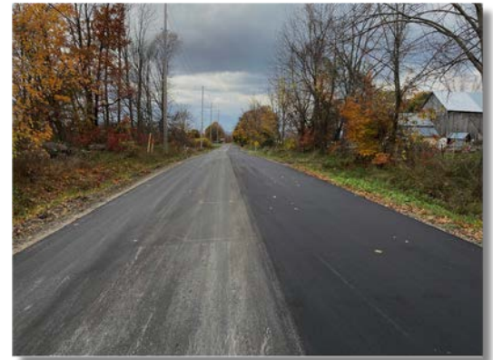
Wood Road at Forgets Road. Paving complete, prior to shouldering.
