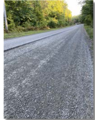
Surface Treatment on one lane at Forgets Road.
