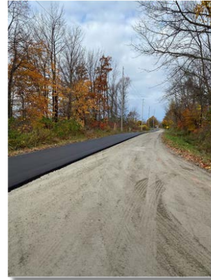
Wood Road at Elliot Side Road. One laneway paved.
