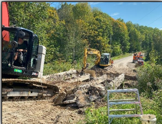
Demolition of the existing bridge
