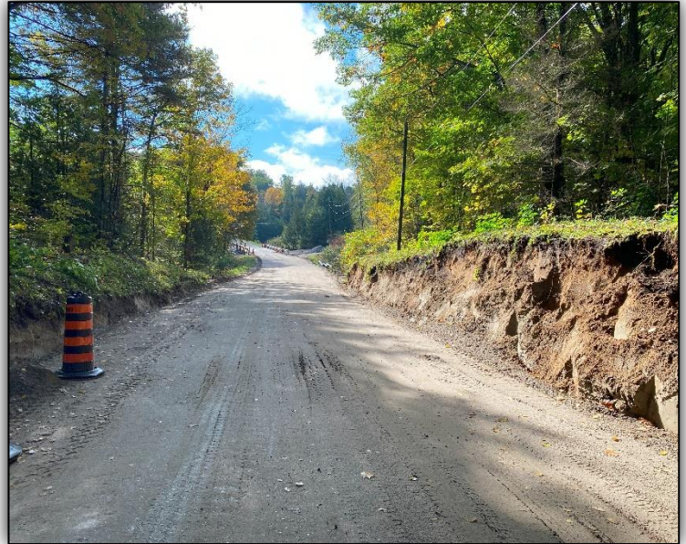
October 2024 – Rosemount Road hill cut in grade, and bend at the bridge widened. This photo was prior to slopes on side of road being cut back.
