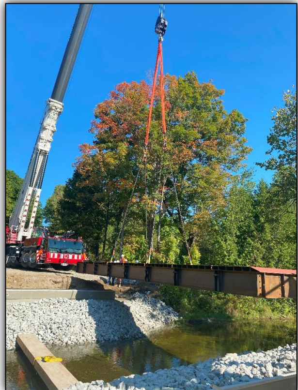
Crane installing a section of the steel bridge deck
