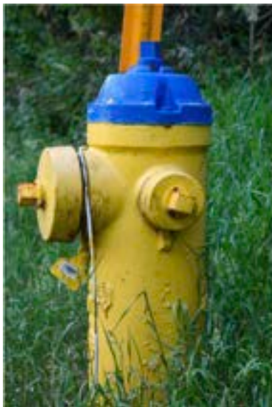
Figure 8. A fire hydrant painted according to the NFPA 291 colour code.
